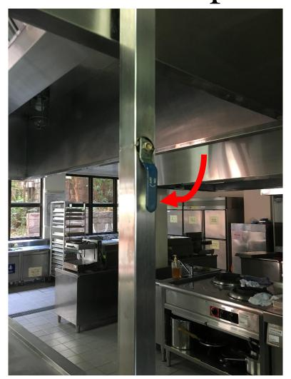
最後: 先把母火轉向開, 再自行決定要用外圈的火或內圈的火。 Final Step: Turn the main fire away and decide on its own to use the fire in the Outer ring or the fire in the Inner ring.
